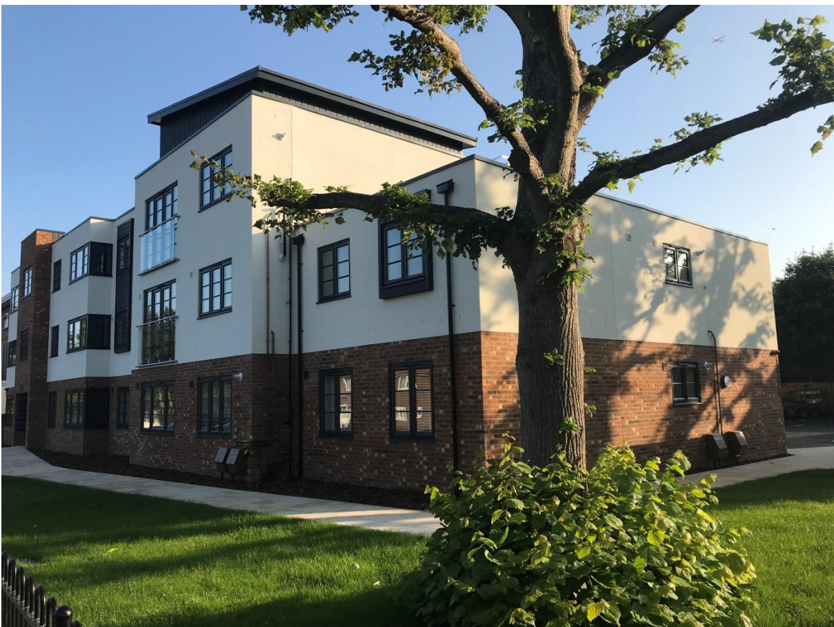
Twin foxes after redevelopment – provision of 14 new council homes in 2018/19
